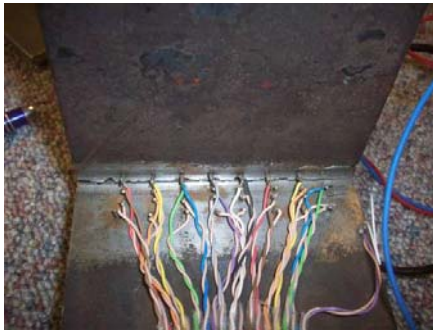
Fig 3a – Electrodes welded along crack site
